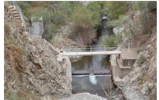
Flow gauging station on Peristerona River near Panayia Bridge. Photo Gerald Dörflinger; date: March 2013
